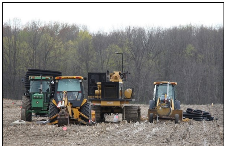
Installation of tile drainage on a farm field adjacent to a woodland.
